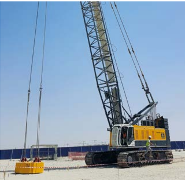
Dubai Creek Harbor, Dubai, UAE Improvement of the construction soil over roughly 500,000 m 2 using vibro compaction and dynamic compaction.
