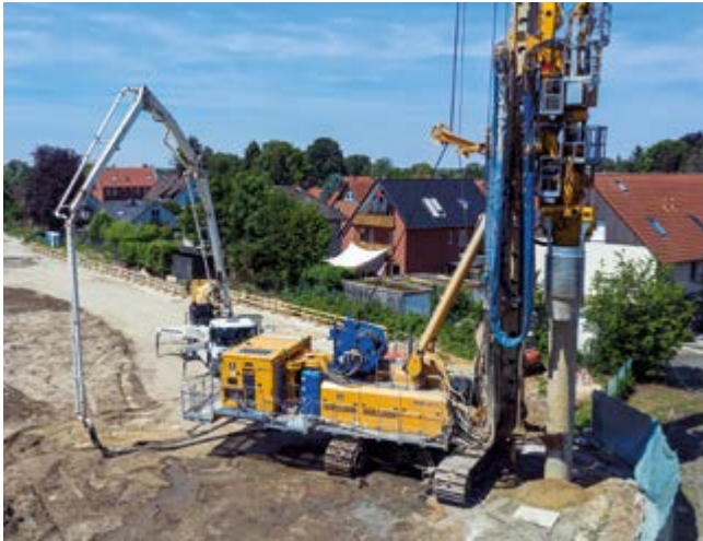
Businesspark, Hannover, Germany Construction of secant pile wall with a diameter of 880 mm and depth of 16 m using the double-head drilling method.
