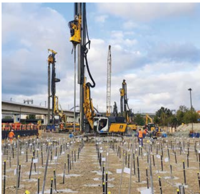
Quartier Heidestraße, Berlin, Germany Execution of 16,000 m 2 of LWS silicate gel base by means of pore injection.
