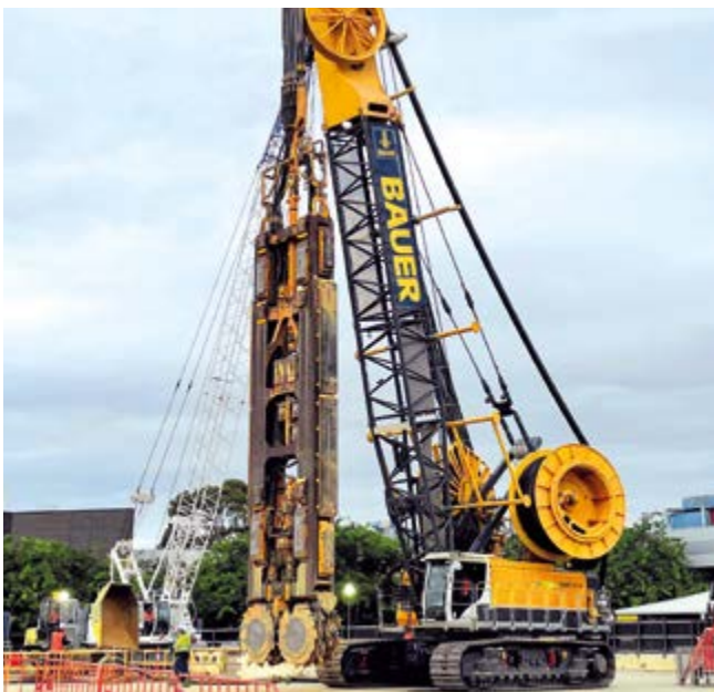
Hobson Bay, Melbourne, Australia Construction of two shafts using an MC 96 duty-cycle crane with a BC 48 trench cutter.
