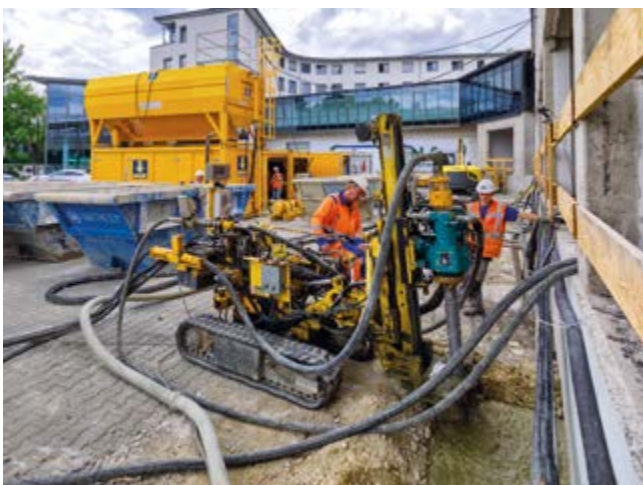
Strengthening the foundation of an industrial building, Munich, Germany As a reinforcement measure, 130 columns were installed up to a depth of approx. 8 m using PI
