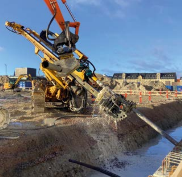
Operaparken, Copenhagen, Denmark Tie-back of a diaphragm wall in two anchor layers with a total of 186 temporary strand anchors.
