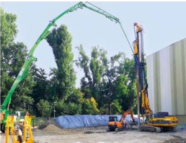
Logistics Center, Karlsruhe, Germany For the foundation work on a logistics center, Bauer carried out 2,700 m of vibro concrete columns.
